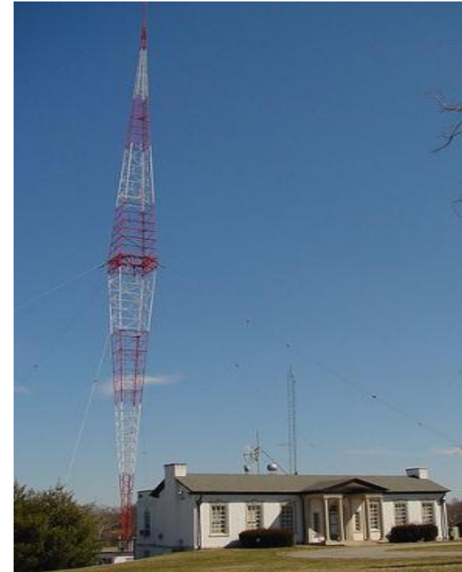
808 Ft Broadcast Monopole WSM 650 AM (erected in 1932)
