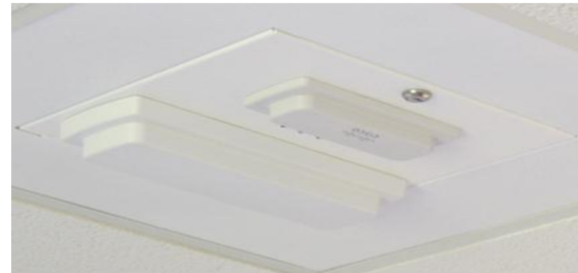
Rugged AP in ceiling enclosure
